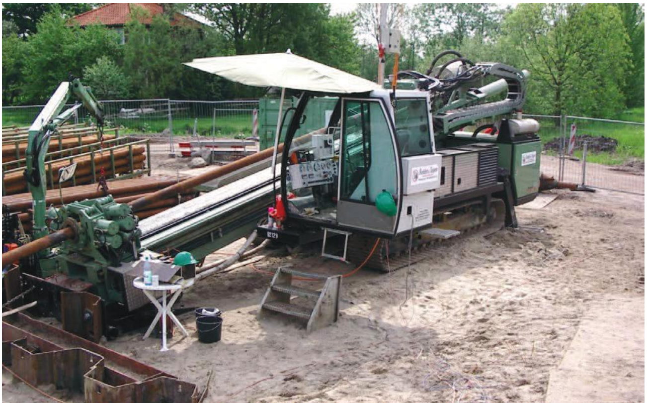
Figure 25. Example HDD rig of the midi size likely to be used for the short HDD's. A sheet piled rig anchor is visible on the left.
