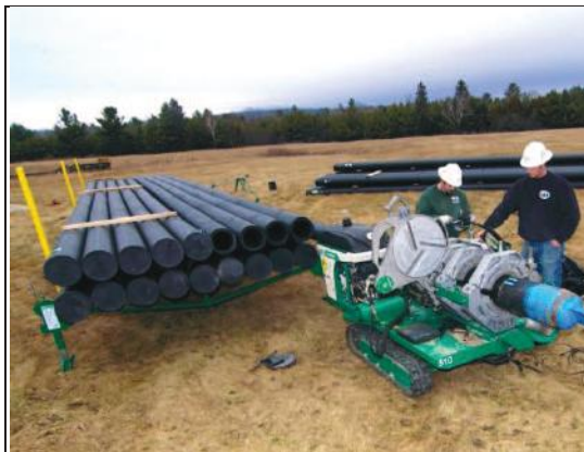
Figure 29. Typical setup of PE butt fusion welder
