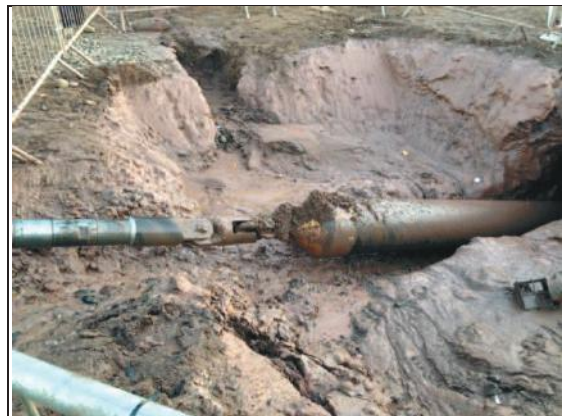
Figure 30. Drilling rod, swivel, pulling head and duct being pulled into the entry pit
