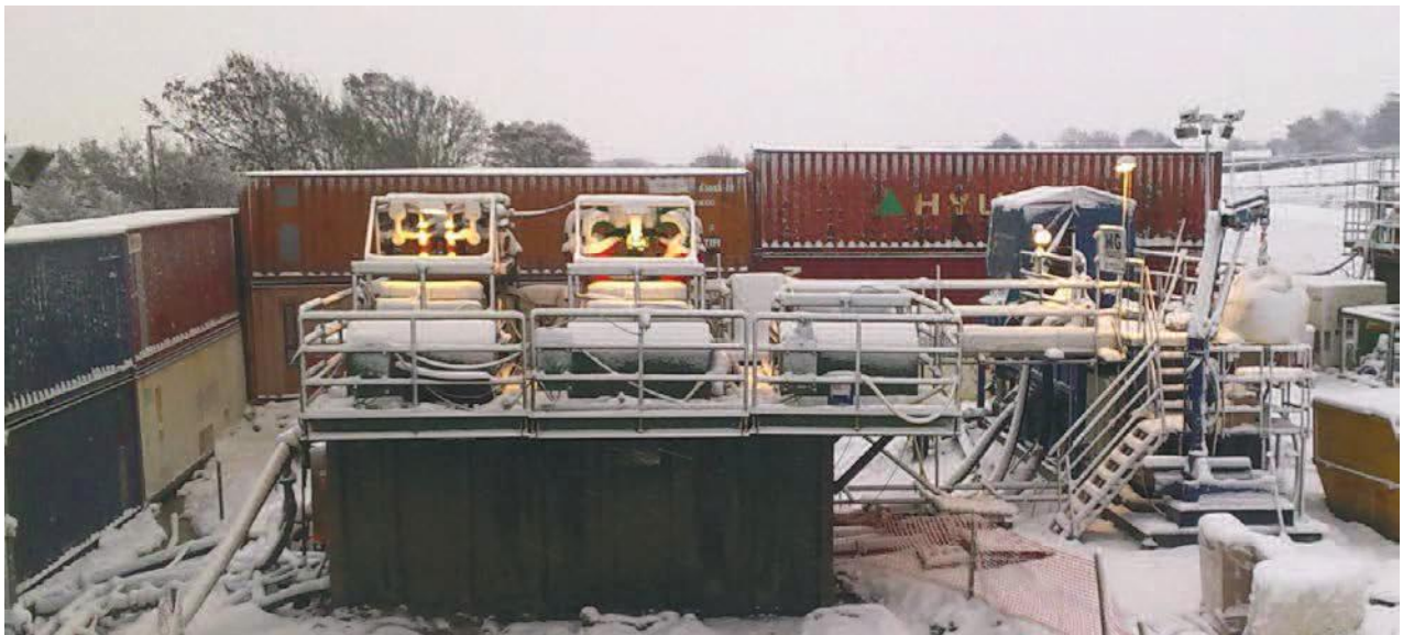
Figure 14. Stacked shipping containers used for noise attenuation panels on a UK project. There were 4 residences within 50m of the site. The work included regular evening work as well as 24hr working during pipeline installation.
