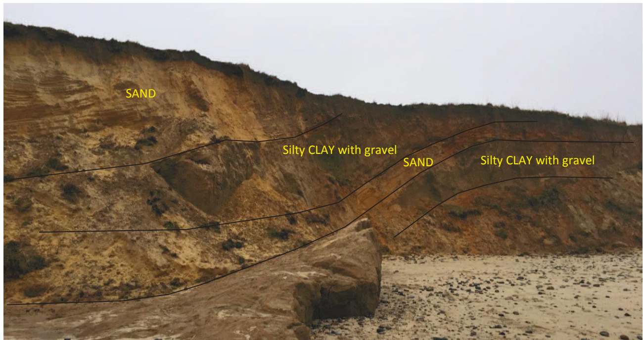
Figure 6. Photograph showing the north-western margin of the subsidence basin. The lower left of the photograph shows the lower silty CLAY with gravel layer within the basin approaching a near horizontal attitude. The right of the photograph shows the horizontal strata in the unaffected zone. The centre of the photograph shows inclined strata along the margin of the subsidence area.
