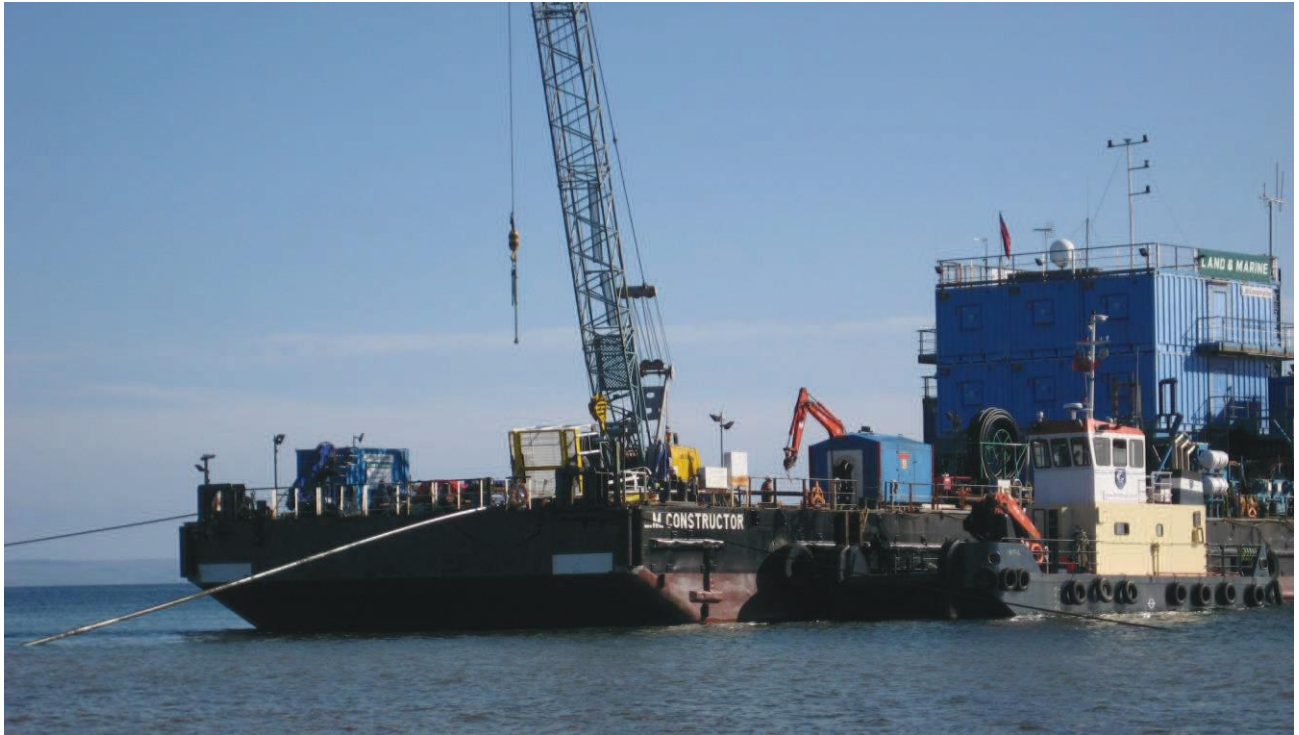
Figure 19. Pilot drilling string being pulled aboard on a UK project after an exit in 5m water.
