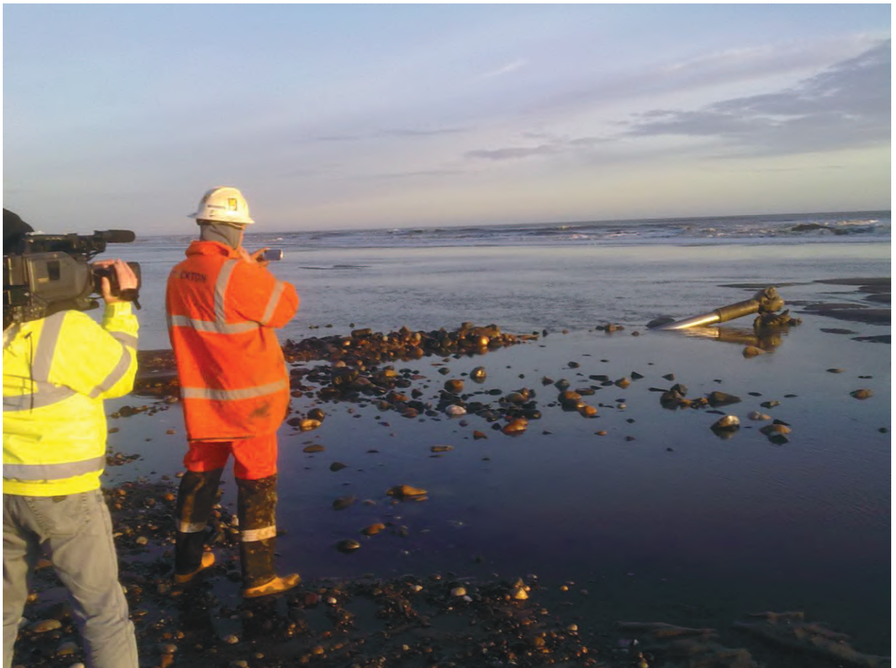
Figure 18. Pilot hole beach exit on a UK cable landfall project.
