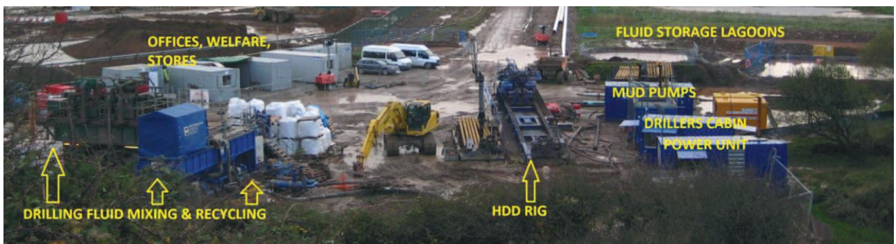
Figure 23. Example HDD site layout. Fluid storage lagoons are sometimes replaced with storage tanks.
