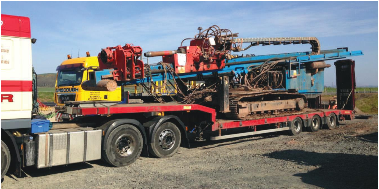
Figure 22. A standard HDD maxi rig being delivered to site.
