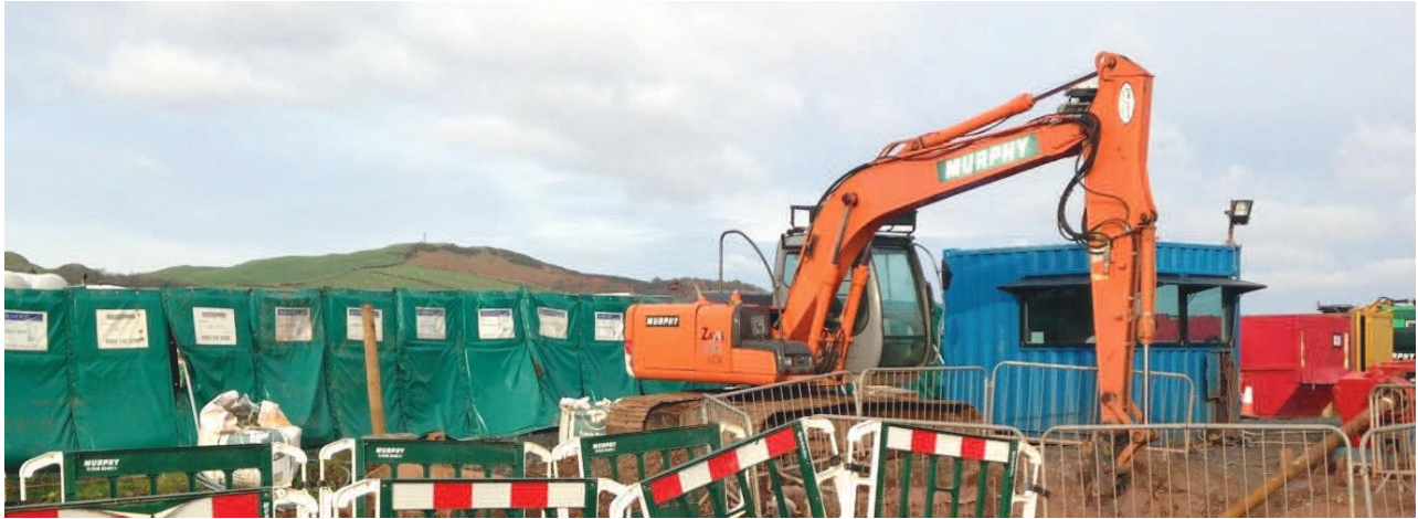
Figure 13. Noise attenuation panels on Heras Fencing on a recent UK project. The nearest neighbour was 100m from the panels. The work included allowance for 24hr working during duct installation.
